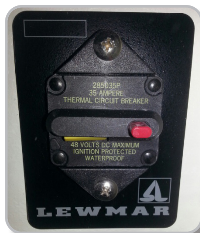
The windlass breaker is mounted in the head/console compartment.
